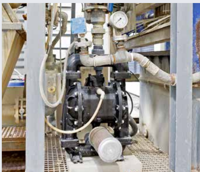
High suction lift reduces pump delivery.
